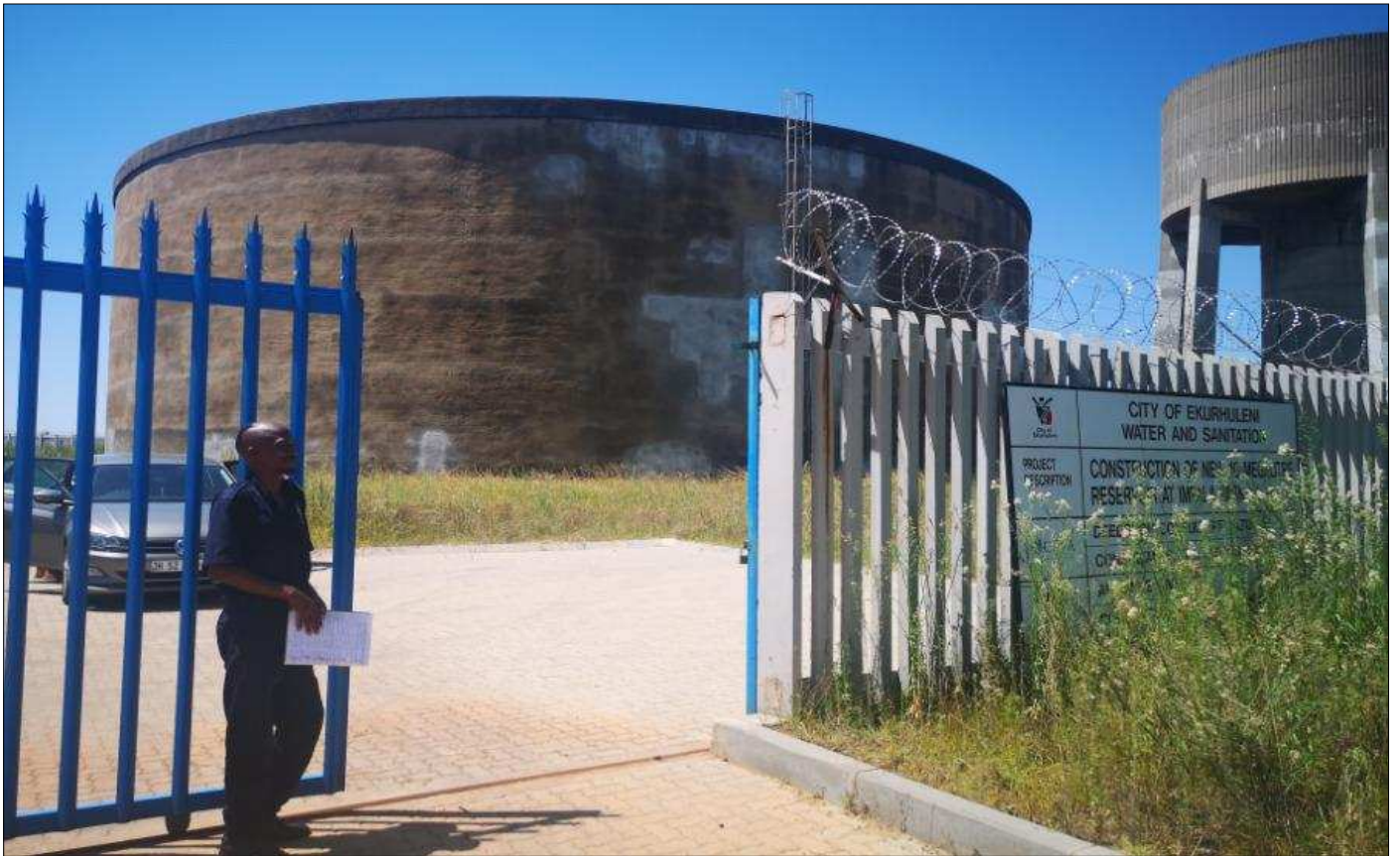
Impala reservoir secured, sign posted, neat terrain
