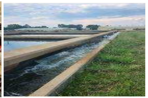
Sedimentation tanks at Balkfontein WTW
