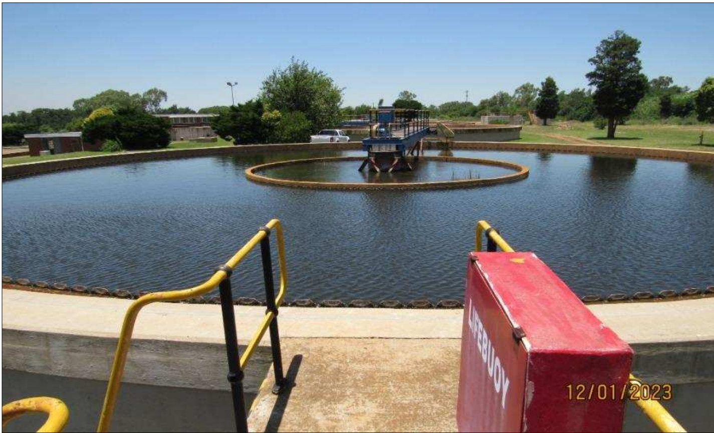
JB Marks: Settling tanks in immaculate condition, cleared of solids, delivering SANS241 compliant water
