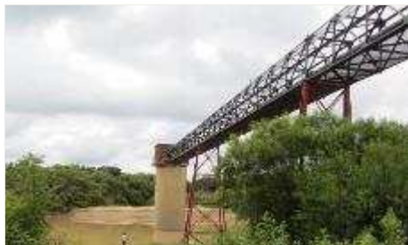
Raw water pump station
