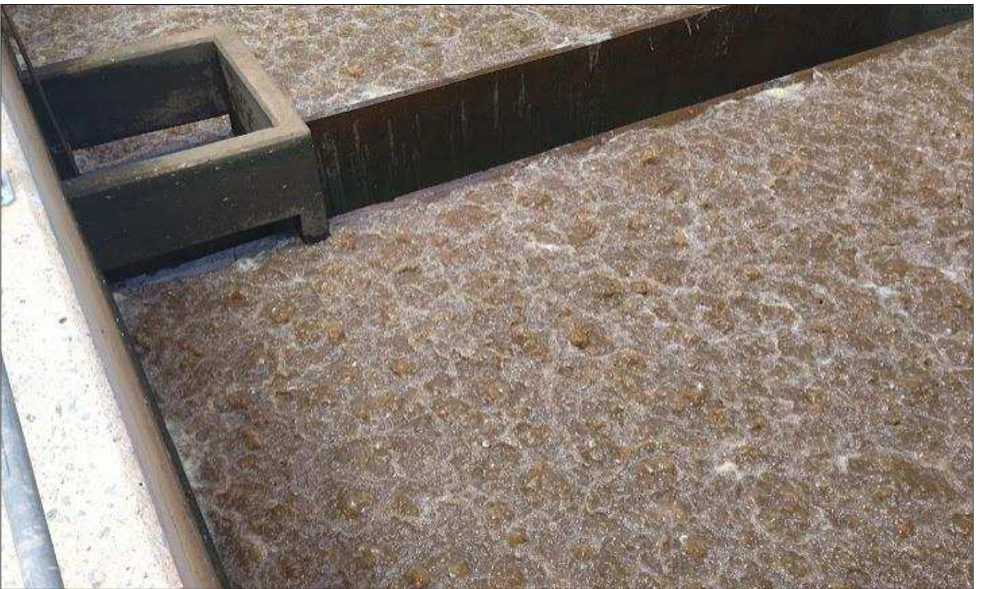
Saldanha: Withoogte WTW filter backwash – true excellence
