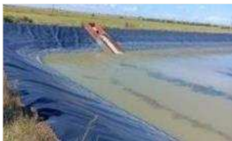
Hertzogville Water Purification Plant`s raw water holding dam and the raw water is abstracted from Vaal River under Water Use License No: - 10/C91A/ACL/1915
