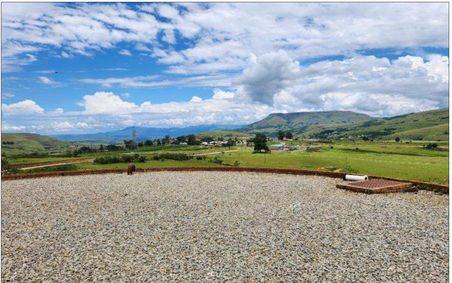
Impedile Town: View from top of reservoir 2, good structural integrity
