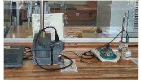
Excellent monitoring equipment at Balkfontein WTW
