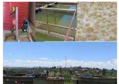
Ficksburg WTW treatment processes
