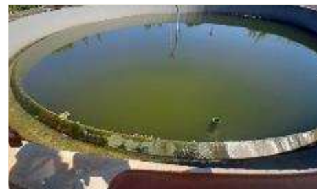
Old settling tank still being used
