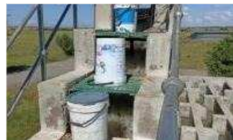
Picture of a typical rapid mixing at Hertzogville Water Purification Plant, a channel with rapid fall in level and buckets with a water treatment chemical liquid
