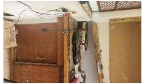
Lack of facilities: There are no toilets or bathrooms on site, office and kitchen has broken furniture and old equipment, Kitchen serves as Lab
