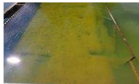
Lamella plates within only a part of the settling tank
