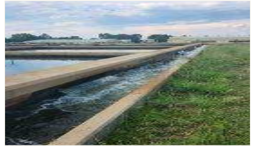
Sedimentation tanks at Balkfontein WTW
