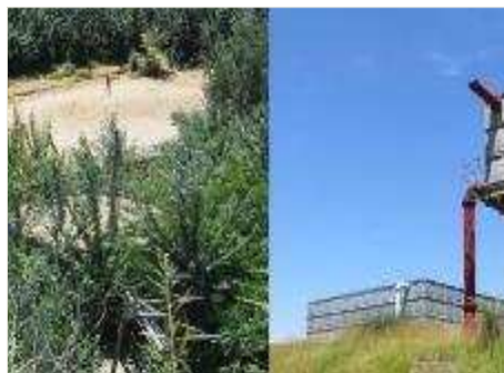
Raw water pump station in Caledon River with two on-site raw water reservoirs receiving water from the Meulspruit and Caledon River
