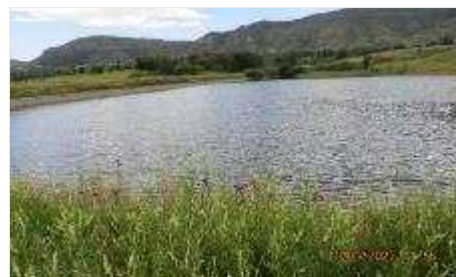
Townsend dam. The Clarens water treatment plant receives raw water from the Caledon River via the Townsend dam
